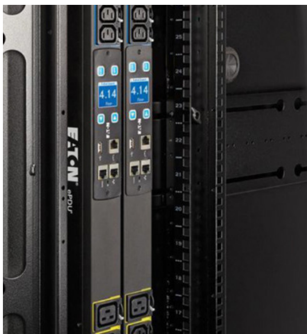
Figure 17-“Smart plug” power strips in cabinet
